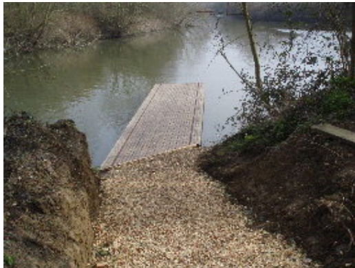
The canoe portage platform downstream of Oak Weir Lock
